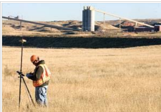
Paul Guajardo, a surveyor for Ames Construction, records positions for a power block that will accompany the new Dry Fork Station power plant. The 385-megawatt plant construction began Wednesday north of Gillette near the mouth of the Dry Fork mine. — News-Record photo by Nathan Payne
