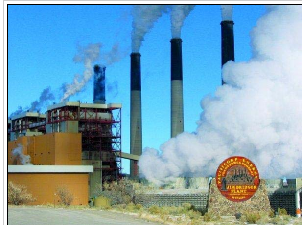
Two expansion projects planned at the Jim Bridger power plant in Sweetwater County have been set aside, PacifiCorp officials say. Star-Tribune file photo.
