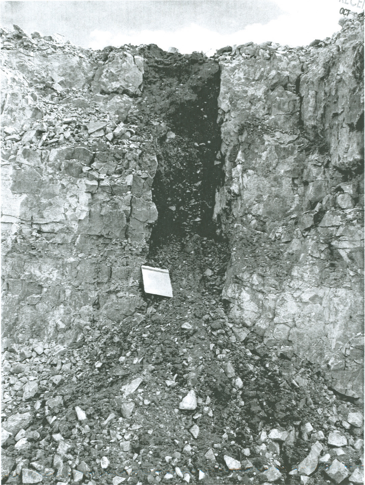
Figure 1. Sand filled fracture exposed at the present surface and now in the wall of Etchepare 7A east of Area "C".
