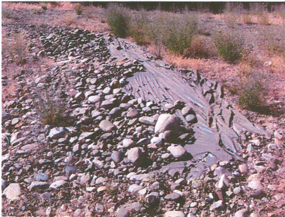
Figure 4 - View of uncovered liner
