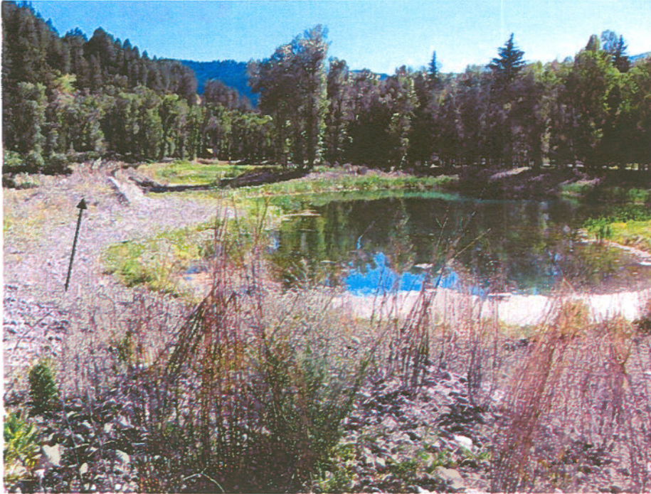
Figure 3 - View S of Pond No. 1 (see attached map). A topsoil stockpile is evident to the left of the pond (arrow).
