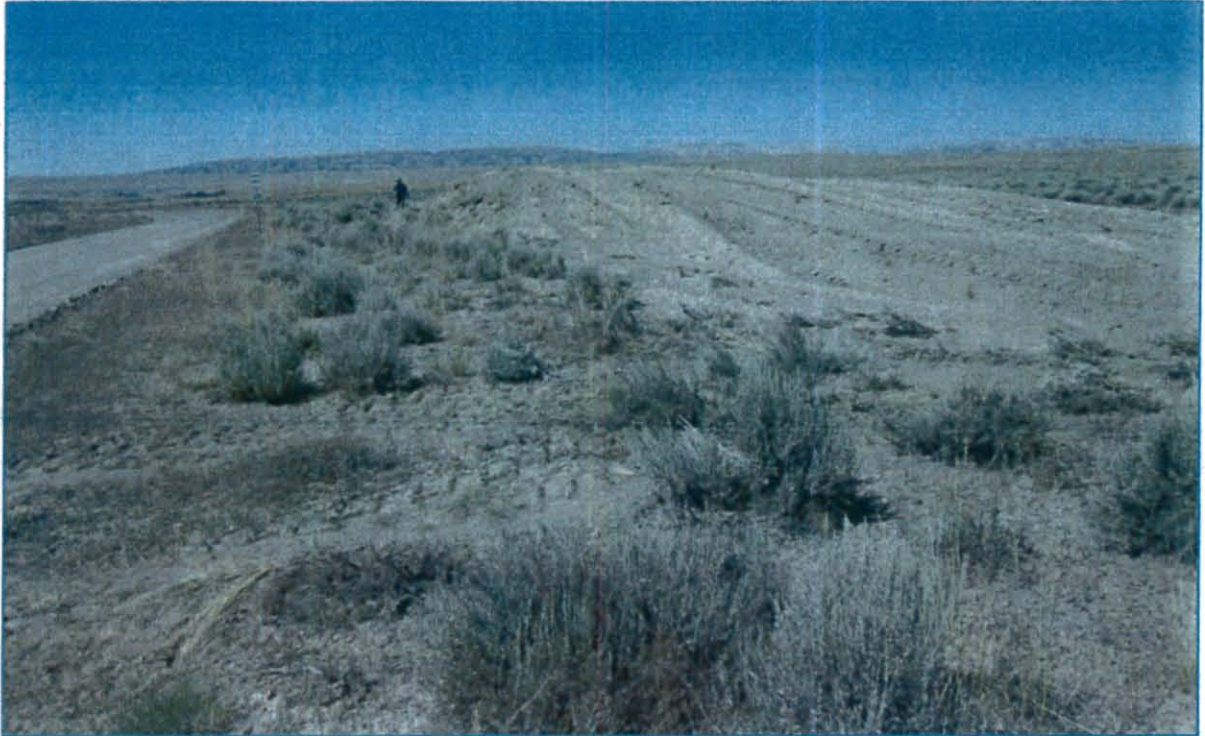
Photo 3 (above) looks southwest and shows the topsoil stockpile that has been constructed adjacent to the Access Road. Photo 4 (below) looks south at the active pit area (boom and bucket of the trackhoe are barely visible just to the right of photo center). Overburden from the initial boxcut has been stacked to the northeast. In the foreground is a windrow of what is construed to be suitable material.
