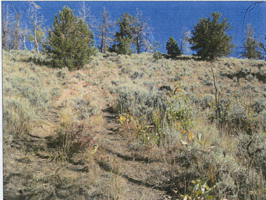
Photo Number 4: This depicts a steep portion of the two-track road leading to the upper three excavation sites dug under Permit 310c. This is one of the several locations along the access route that is in need of a water bar.
