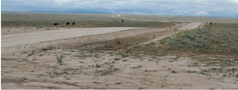
a) Intersection with Wamsutter/Crooks Gap Road, facing north.
