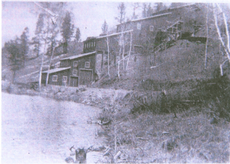
The Mineral Hill Properties mill facility above Spotted Tail Gulch as it appeared in 1935. The facility was designed as a 200 ton per day mill.
