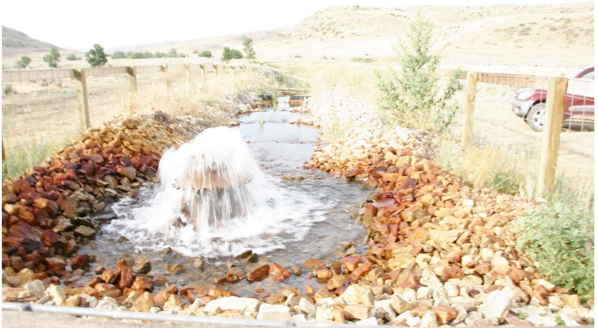
Discharge location to reservoir on Cat Creek.
